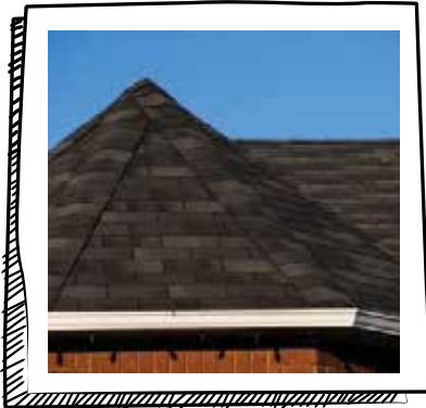
ADDING THE ROOF
