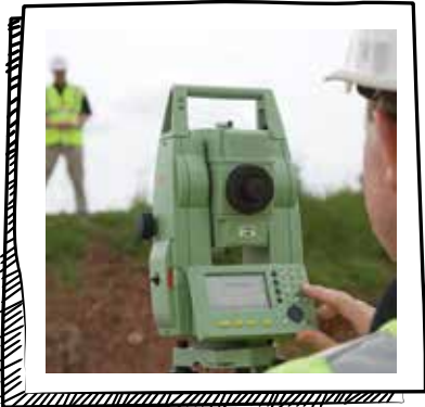
SURVEYING THE SITE
