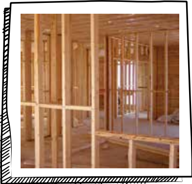
ERECTING THE WALLS
